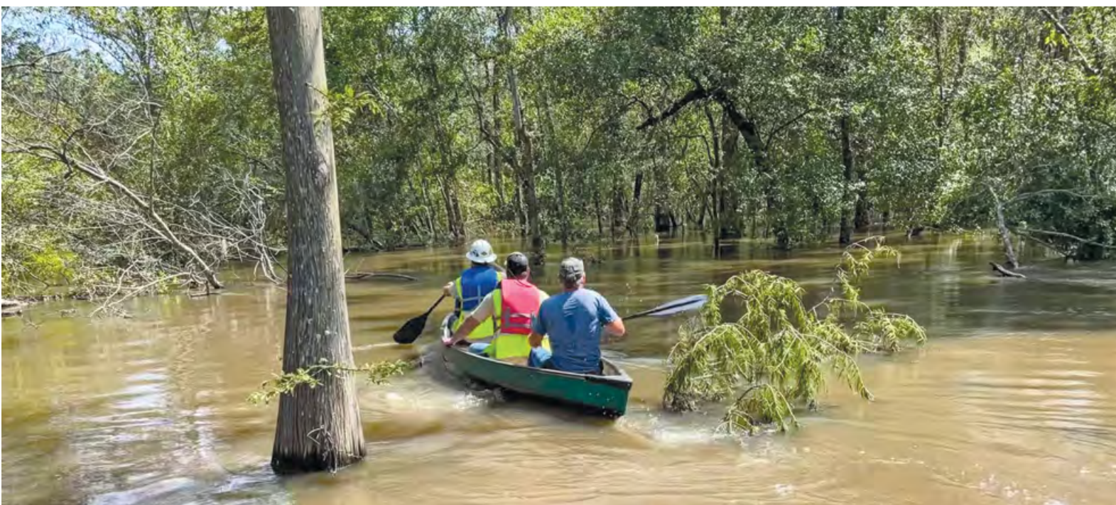
At left: Restoring power in the Bayou included a canoe trip for Louisville Local 2100 foreman Travis Garrison and his crew, who were vigilant about avoiding alligators and other swamp creatures.
